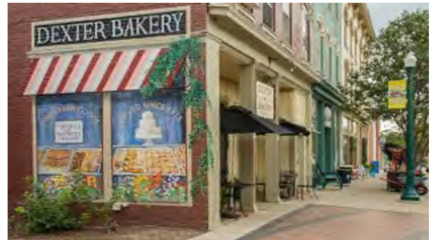
Street Wall Maintained with Inset Dining
